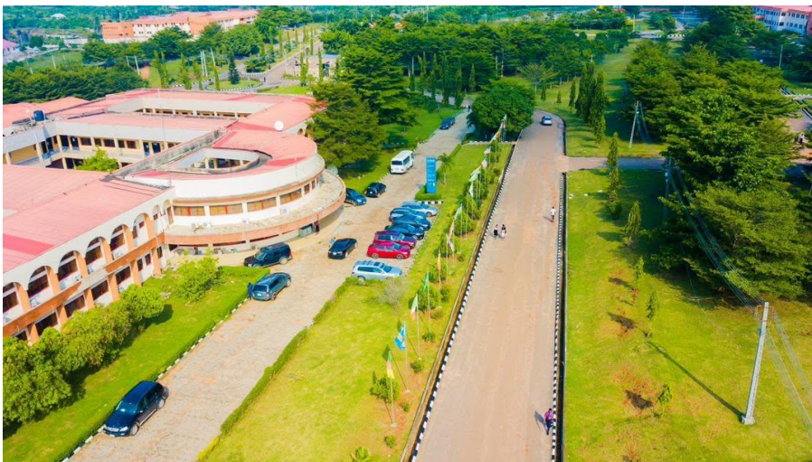
Plate 3.1: Aerial View Of Caleb University Administrative Building, Imota, Lagos State
