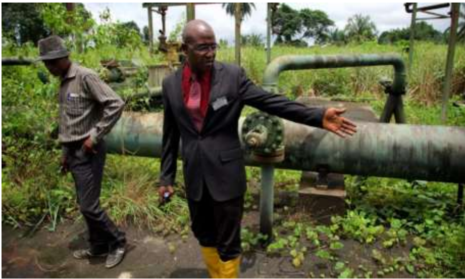
Plate 2.2: Official of inspecting oil spill sites in the Niger Delta
