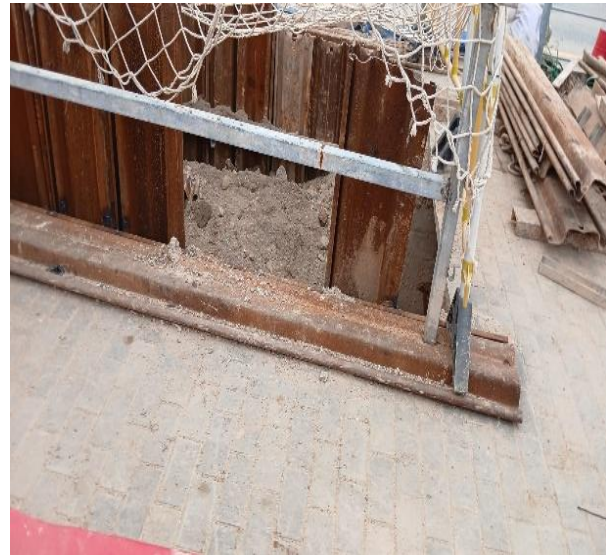
Figure 4: Barrier is fixed by metal trunking
