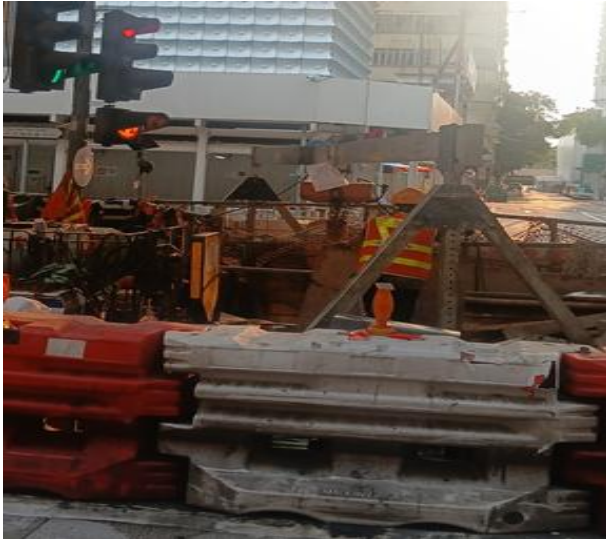
Figure 3: A frame with winch is set up
