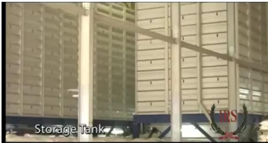
Plate XV: IRS rice milling factory Kano Storage tank
