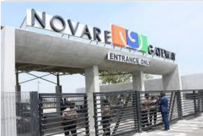
Figure 4: Approach view of Novare Gateway Mall
