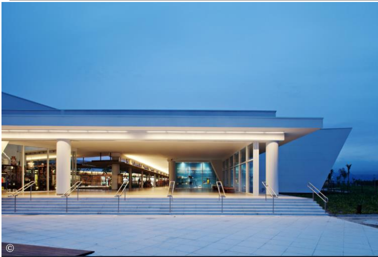
Figure 8: Approach view of serramar paque mall
