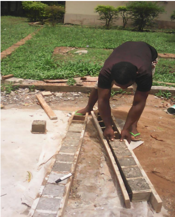
Figure 6: Dismantling the mold frame after CCH concrete is hardened
