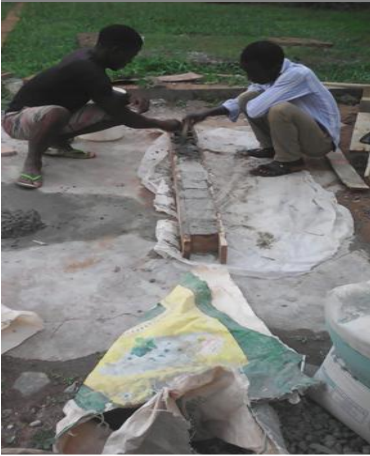
Figure 5: Moulding CCH cubes using wooden frames
