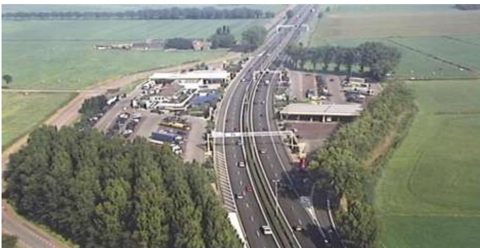
Figure 2: Aerial photo of the De Lucht Rest Area along the A2 Holland: Source: Dennis, (2019)
