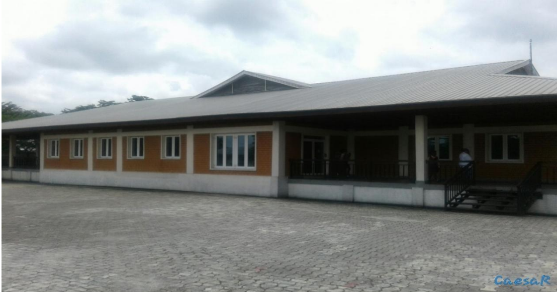
Plate 1: Approach view of the Appropriate Technology Enabled Development (A.T.E.D) Demonstration Centre Building (source; Researcher's field study (2023)).
