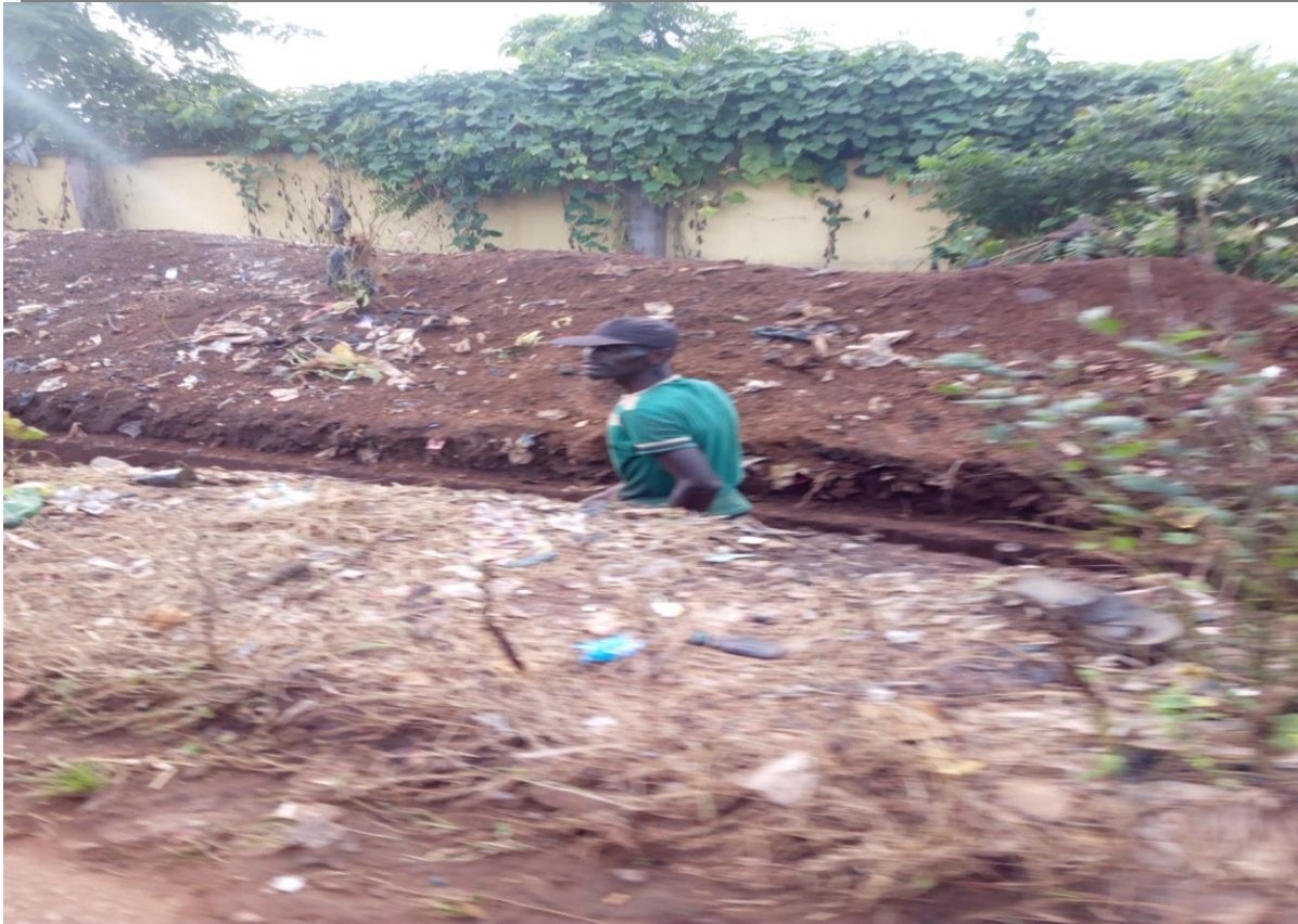
Plate 2: Evacuation of drainage channel for easy flow of run-off water
