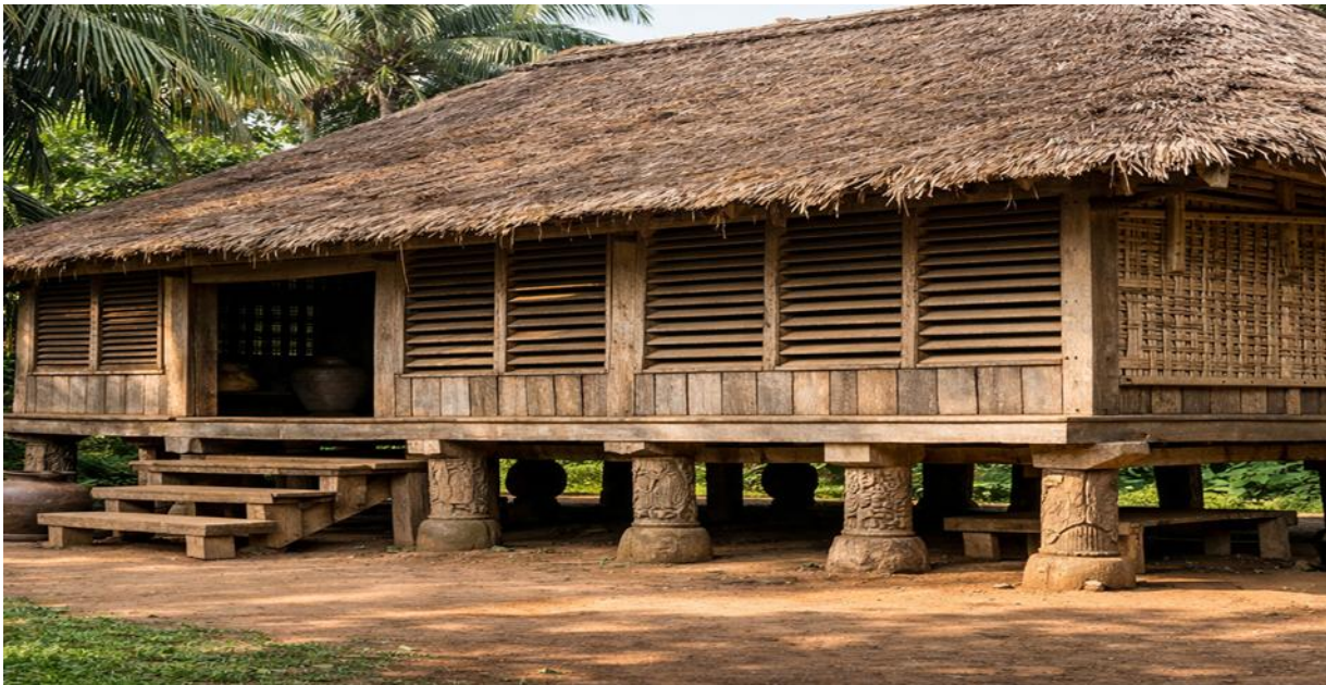
Figure 2. Natural ventilation features: louvered screens and elevated floors in southeastern Nigeria
