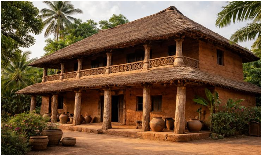
Figure 3. Traditional Nigerian mud and timber building with high thermal mass walls in southwestern Nigeria
