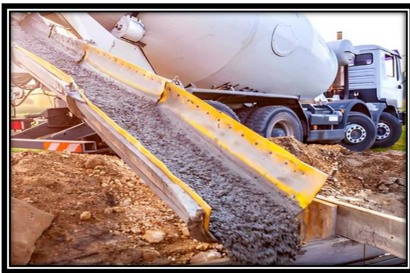
Figure 9: Granite Mixer in a Construction Site
