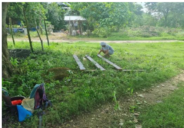
Figure 5.21. The assembling of the signage in the Sendong signage in the Sendong Memorial Park Photo taken: May 11, 2022
