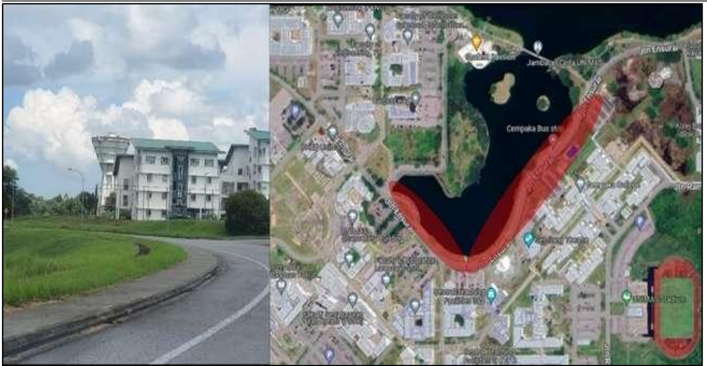
Figure 3: Pedestrian walkway (sidewalk) near road and next to UNIMAS lake
