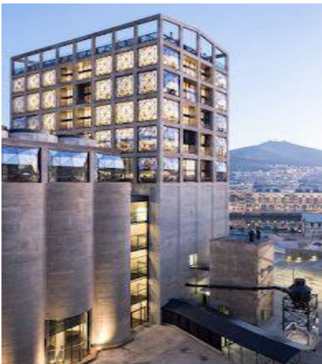
Fig 8: showing fritted glass façade (Source: archdaily.com)
