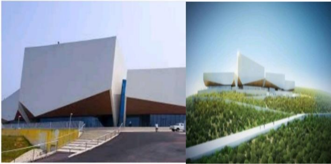
Fig 4.2: Picture of Exterior View of Calabar International Convention Centre.
